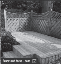
Fences and decks – done
